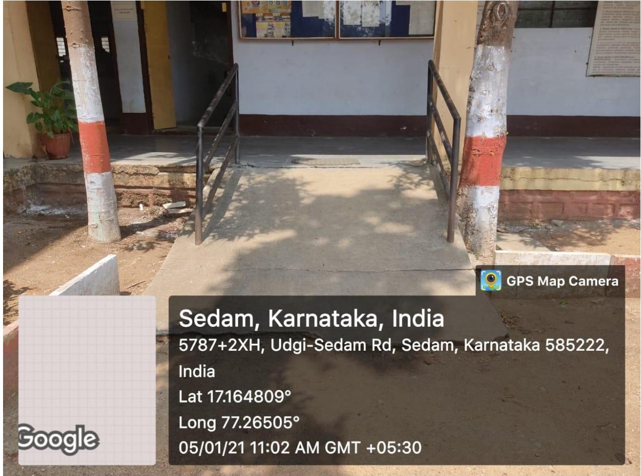
RAMP for Disabled
